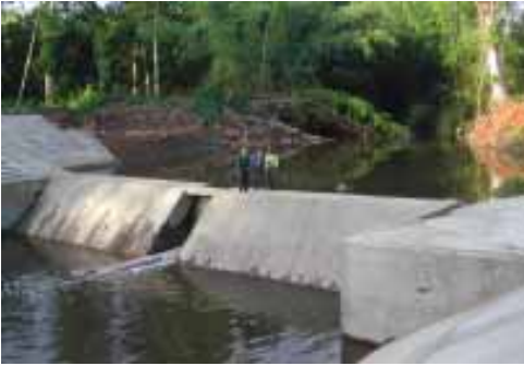
A dam in Yok Don National Park built to provide water resources for wildlife in the dry season.
